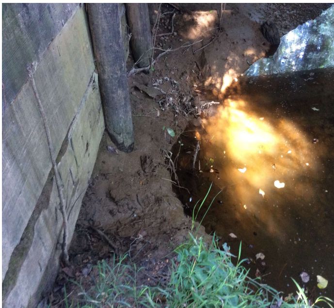
PHOTO 1 Description Abutment 1 right side erosion.
