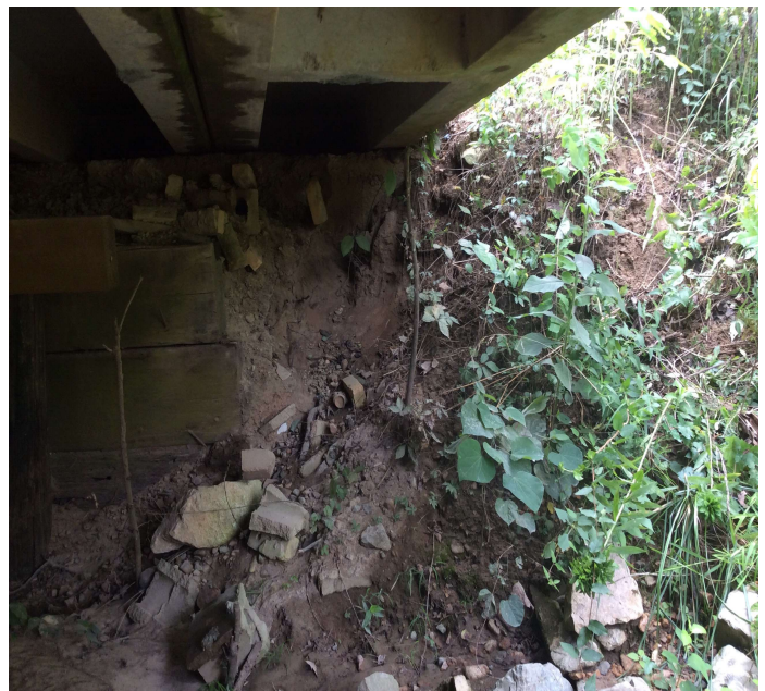
PHOTO 2 Description Abutment #1 left side erosion
